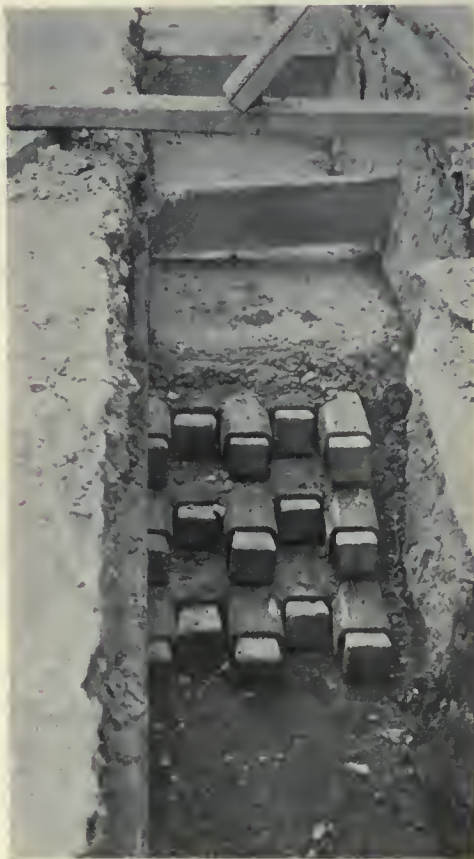
15 duct run showing concrete encasement.
